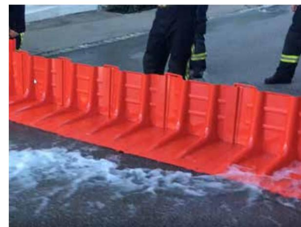
During an exercise, the flood protection system was already set up and withstood even directly approaching water. This means that accumulation heights of 50 cm are possible.
